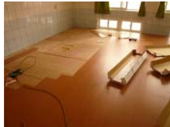
Repairs in progress
