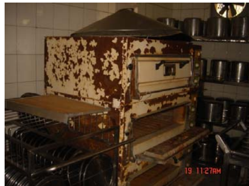
Damaged kitchen facilities
