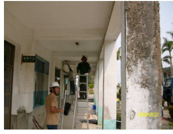
Repairs in progress
