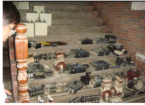
Inspection of dismantled electrical components
