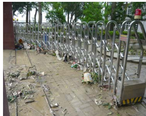
A school gate washed out of place
